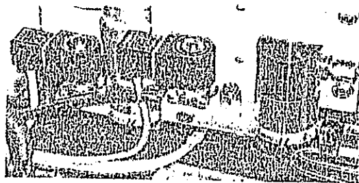
B-DRAIN automatic condensate drain system
